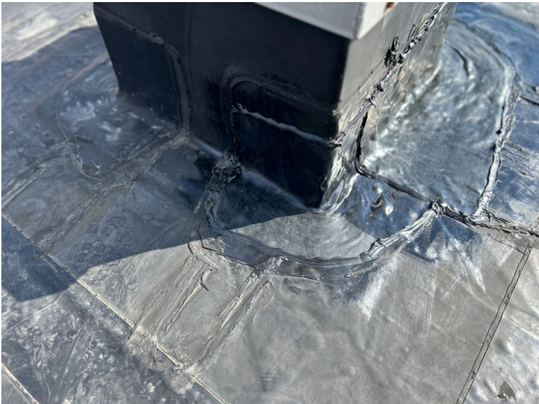
Pictures taken after repairs where made._2
