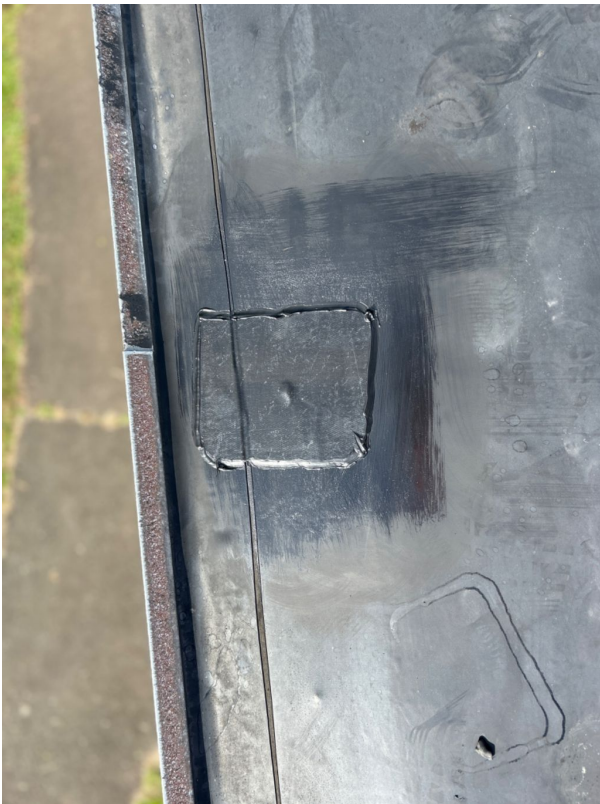
Pictures taken after repairs where made._3
