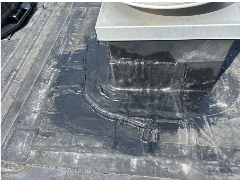
Pictures taken after repairs where made._4
